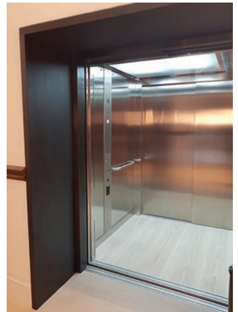
Stainless steel internal finishes with flooring to match the contemporary building design
