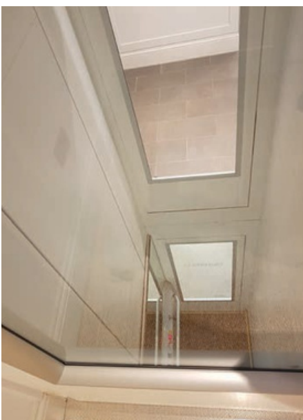
A modern, two stop platform lift installation, specified with glass doors for maximum visibility
