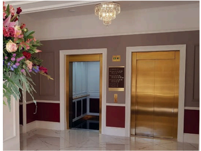
Two passenger lifts installed by Landmark Lifts in the hotel reception
