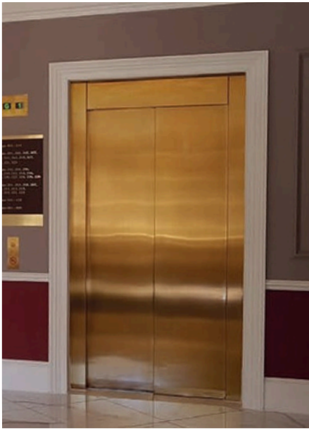
Three bespoke passenger lifts finished with brushed gold stainless steel landing doors
